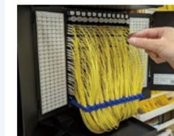
Densely packed optical cords make it difficult to insert and remove connectors
