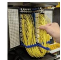
The use of a sliding mechanism for connector trays increases the number of fibers that can be inserted without making maintenance more difficult
